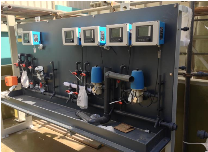
PVC Panel Board for chemical applications
