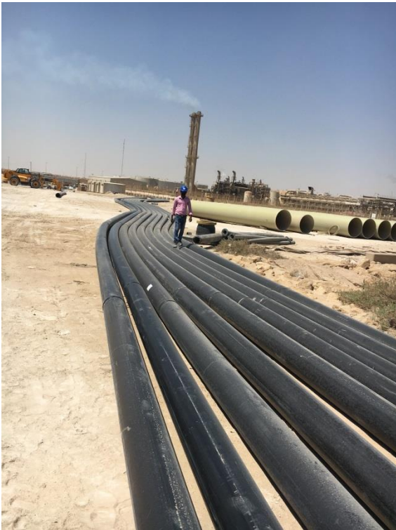
HDPE Pipe installation near Kafji Border For marine applications
