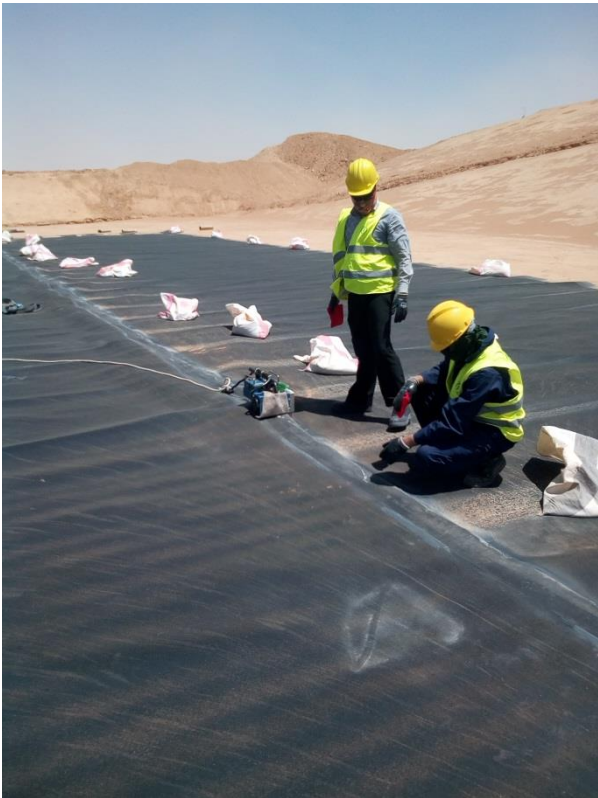
Supply & Installation of HDPE liner in Leaching pads
