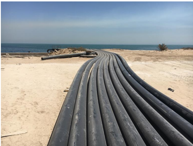
HDPE Pipe installation near Kafji Border For marine applications
