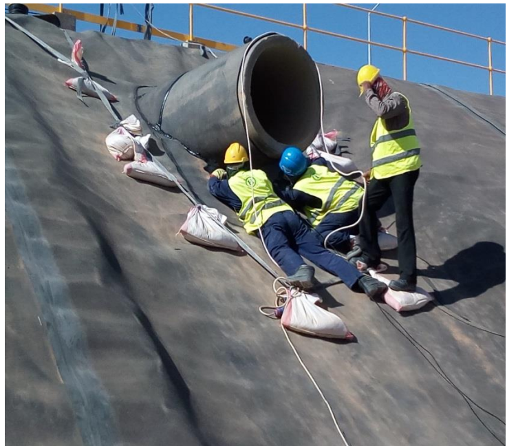
Supply & Installation of HDPE liner in Leaching pads
