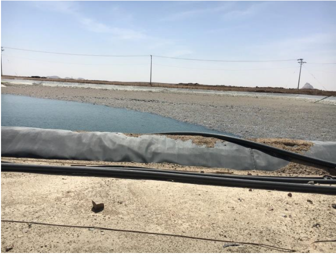
Supply & Installation of HDPE liner in Leaching pads
